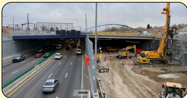
Image 26. Construction of the Lowered Eastbound I-70 Lanes
