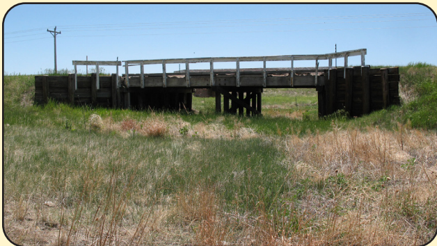
Image 28. I-70 Service RD over Draw in Arapahoe County (F-20-L)
