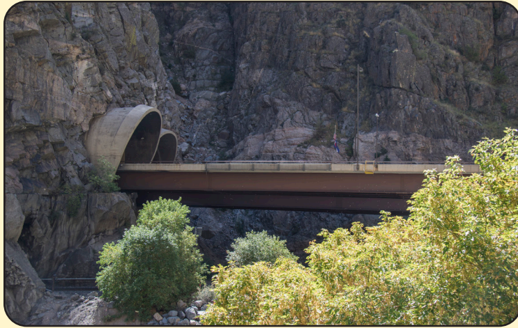
Image 1. Hanging Lake Tunnels in Garfield County
